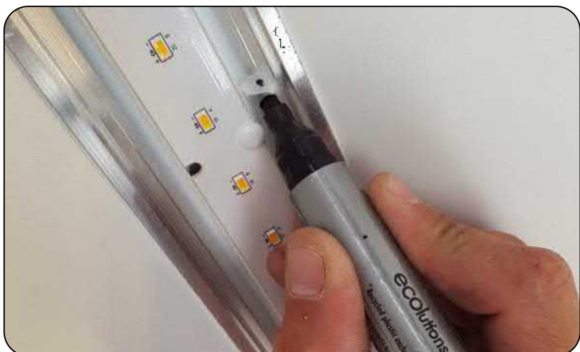
**STEP 3 :** Make the holes for fixation (use a drill if necessary). Place the supplied spacers, where necessary, at the positions of the mounting holes between the profile and the ceiling/wall. The position and the number of spacers needed are determined in function of the state of the ceiling/wall. Attention: after installation the profile may not be bent due to unevenness in the ceiling/wall.
