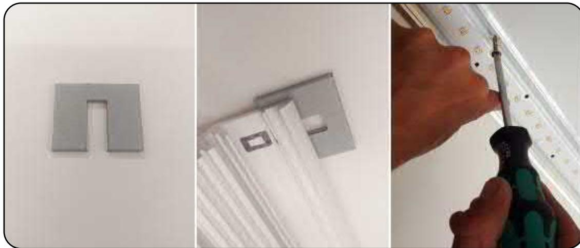
**STEP 4 :** With an internal driver, the terminal is next to the cable entry. Connect the wires and power supply. Pay attention to the colour codes of the wiring: L=brown, N=blue,  $\text{L}^+$ =yellow/green. In case of multiple circuits, regard the colour codes as shown on the wiring scheme (black, orange, grey, red, white).
